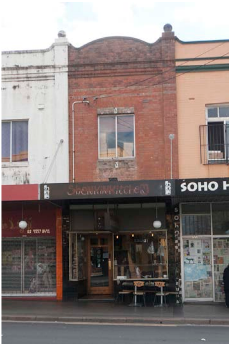
Figure 51: 129 Enmore Road – Federation period shop, part of a simple retail building at 127-131 Enmore Road containing 3 shops. As the façade brickwork to this shop is unpainted, - showing where the door opening has been bricked up below the modern windows to the 1 st floor - this evidence, combined with the original highlight windows above the 1 st floor window to No. 127 (visible at right), reveals the loss of a post-supported balcony to the building. Note recessed entry to ground floor shopfront, which indicates an early shopfront.
