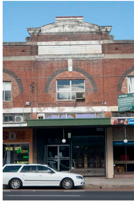
Figure 6: 334 Parramatta Road Stanmore – a contributory building within HCA 5 in the same terrace row as No. 330, retaining face brickwork with stucco detailing to parapet, and with evidence (original brick arch with brick infill and modern windows) for a recessed 1 st floor balcony.
